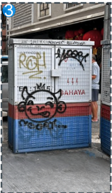
Vandalised TNB feeder pillar
