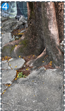
Walkway conditions: Tree roots damages floor (trip hazard)
